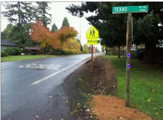
Above: Brown Rd. N.E. - design of sidewalk & bike lanes near Scott Elementary School
