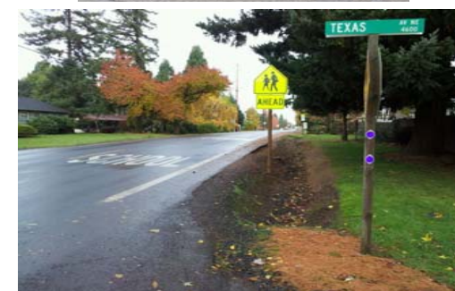
Brown Rd. NE: design of sidewalk & bike lanes near Scott Elementary School (east Salem)
