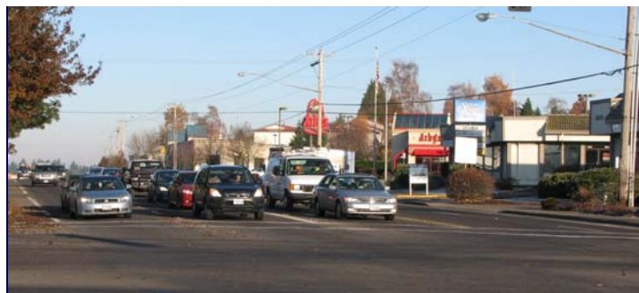
Add dual left-turn lanes for southbound and northbound Commercial St. intersection with Kuebler Blvd. (south Salem)
